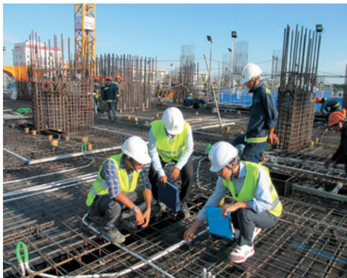
鉄筋結束の技術指導 / Technical instruction for binding wire
