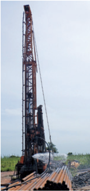
井戸掘削リグの洗浄場水作業 / Well drilling rig in pumping and washing works
