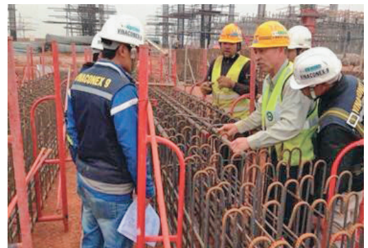
鉄筋工事の技術指導 / Technical instruction for wire binding
