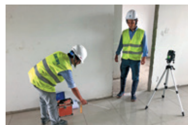
測定の技術指導 / Technical instruction for surveying SORA garden I
