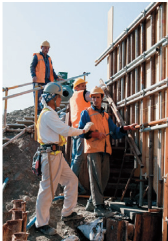
型枠作業指導 / Technical instruction for formwork
