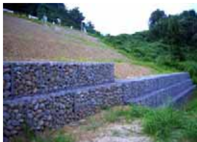
< 盛土のり尻補強 >
