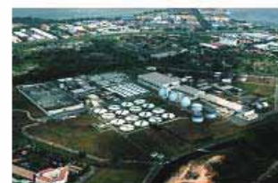
WWTP in Singapore (75,000 m 3 /d)
