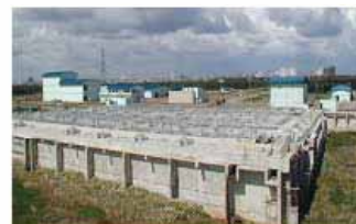
WWTP in Vietnam (141,000 m 3 /d)
