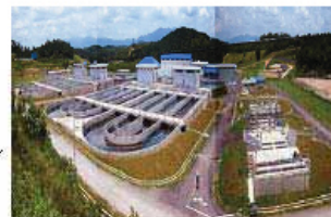
WWTP in Malaysia (59,000 m 3 /d)
