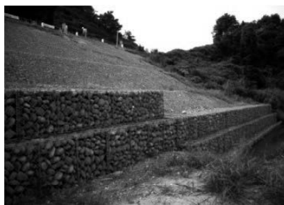
< 盛土のり尻補強 >
