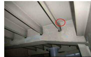
鋼床版のき裂
