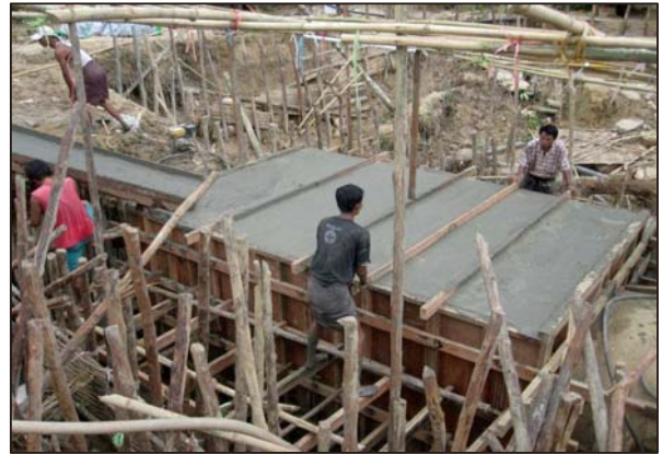
CONCRETE ANCHOR BLOCK
