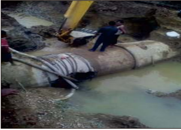
EXCUVATION FOR PIPE REPAIRING
