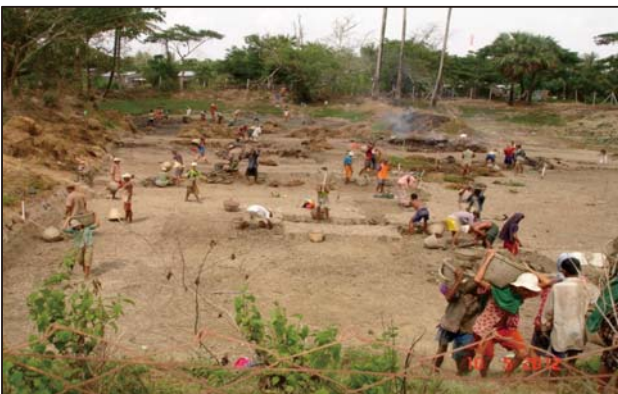
REHABILITATION OF LAKE
