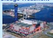
Centralized Sludge melting treatment
