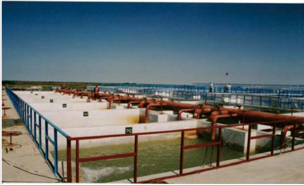
SEDIMENTATION TANKS OF WATER TREATMENT PLANT
