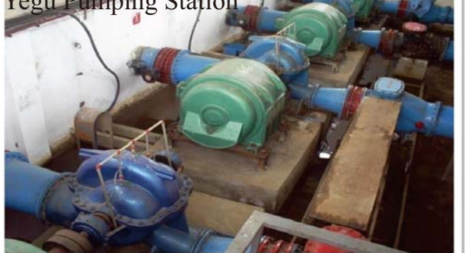
Yegu Pumping Station
