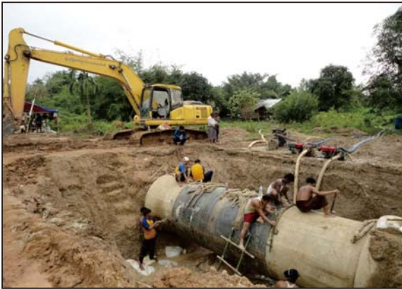
WELDING AND PACKING WITH LEAD AND JUTE
