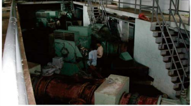
Phugyi Pumping Station
