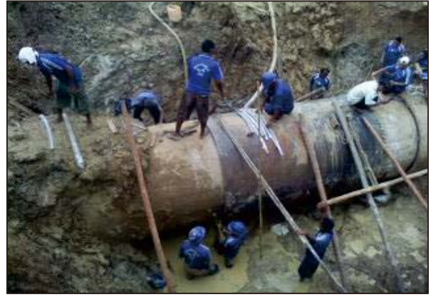
INSTALLATION OF COLLAR
