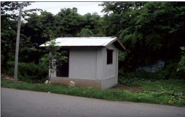
SMALL PUMP HOUSE
