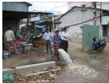
Water pressure check
