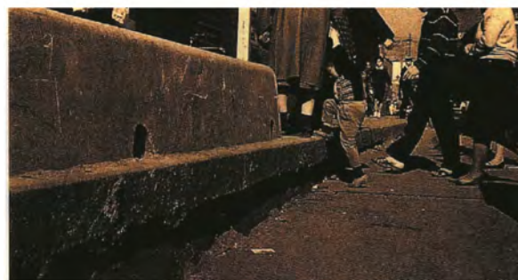
Road Affected by Land Subsidence (Courtesy of Osaka Municipal Waterworks Bureau)
