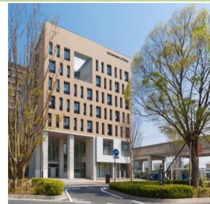
University of Tokyo Kashiwa-no-ha Campus Station Satellite
