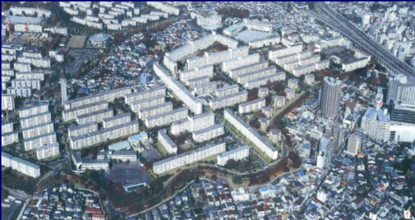
Akabanedai (Before rebuilding, 5 floors)
