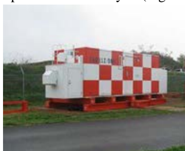
Figure 2.5.2 [Installation of equipment]
