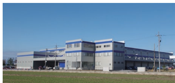
Figure 2-1-91 Exterior of Hakusan No.3 SCM
