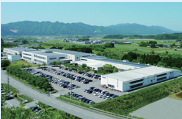
Figure 2-2-54 Niigata JAMCO Production Plant
