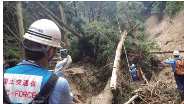
Emergency inspections on sediment-related disaster danger sections (Hiroshima City, Hiroshima Prefecture)
