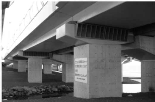
< 橋梁の耐震補強 >
