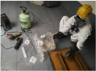
Packing of asbestos-containing material (ACM) in special bag
