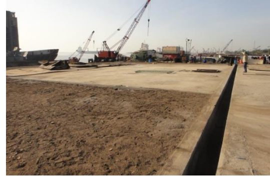
Impermeable floor and drainage system
