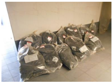
Double bagging of ACM
