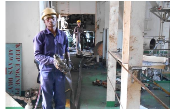
Firefighting found ready inside the engine room
