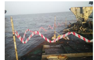
Guard rail for fall prevention from height
