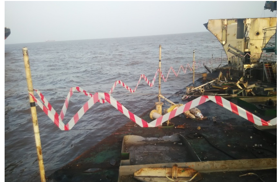
Guard rail (iron wire rope) for fall prevention from height
