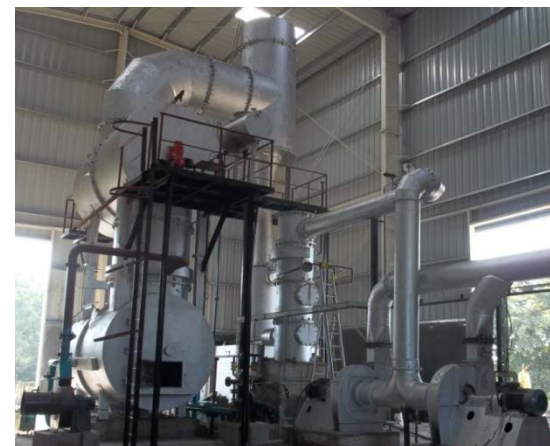
Incinerator at Alang TSDF
