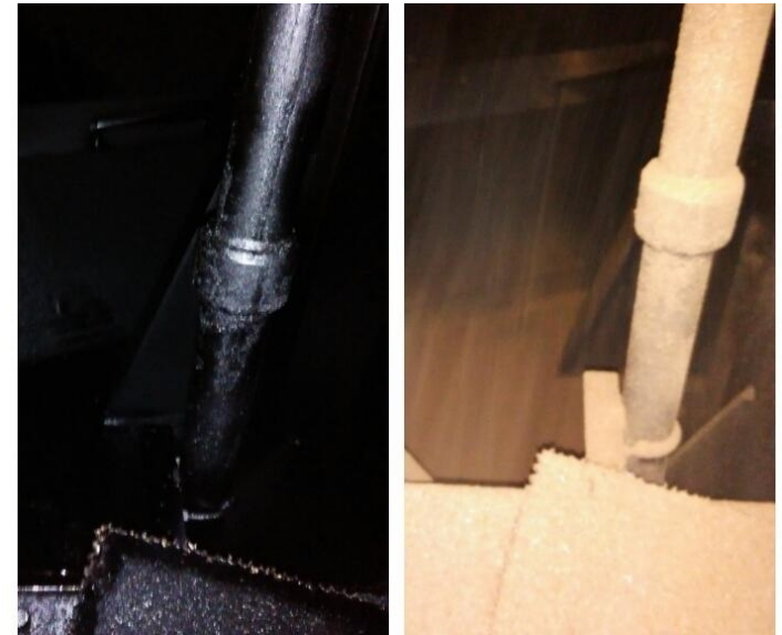
FO Tank before & after cleaning with saw dust
