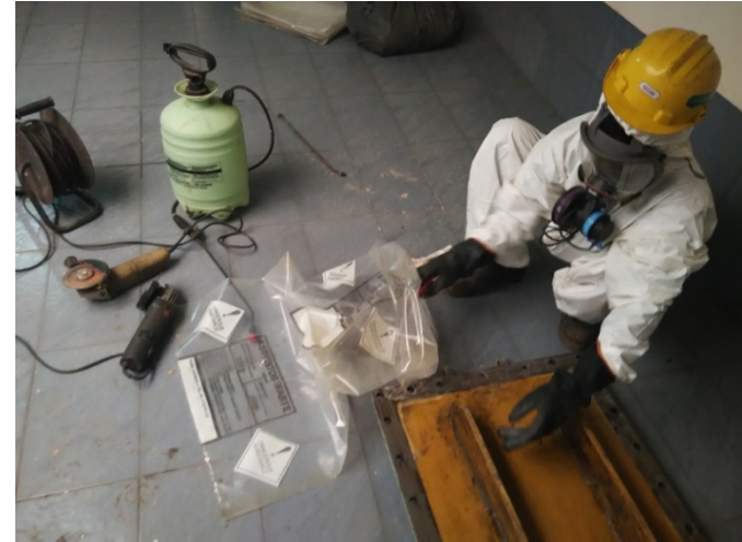
Packing of ACM in special bag
