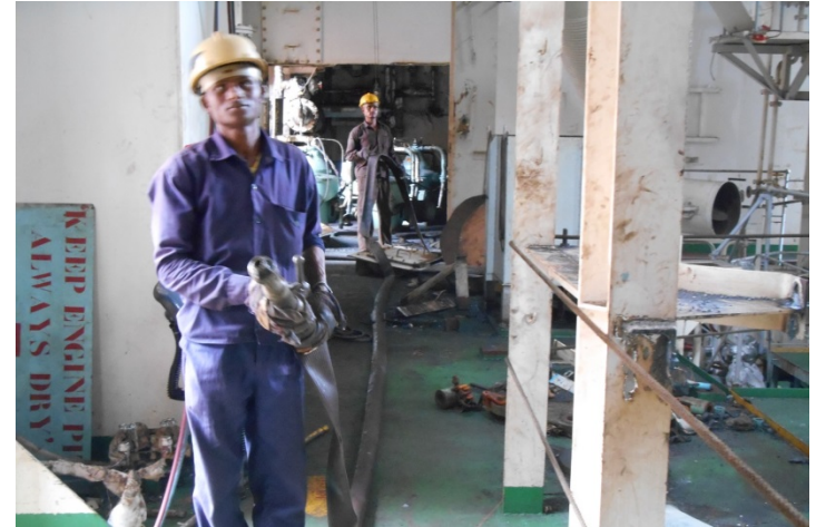
Firefighting found ready inside the engine room
