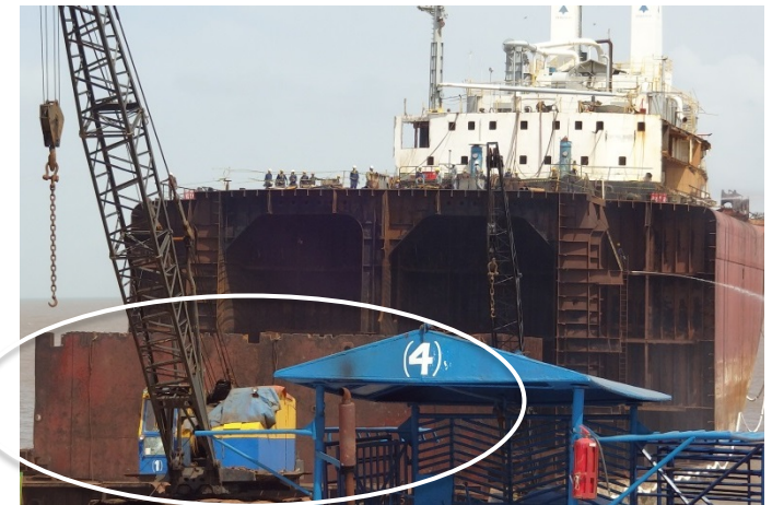
Controlled block falling process
