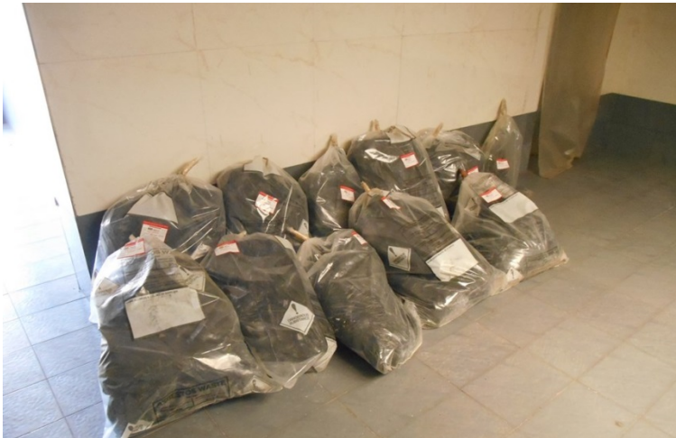
Double bagging of ACM
