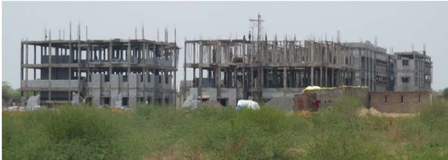
Under Construction Workers' Barracks as in April, 2015 (source: GMB)
