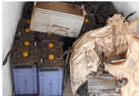
Lead acid batteries
