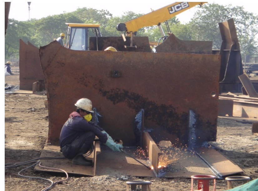
Gas cutting worker with PPE
