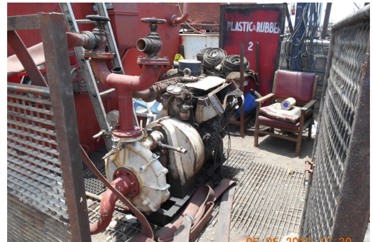
Fire pump on shore
