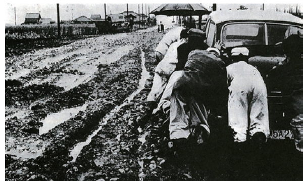
Deteriorated Roads Conditions in 1950s “Watkins Commission Report”
