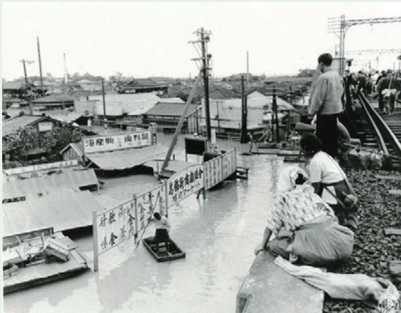
Photo 1: Katsushika-ku experiences flooding up to the eaves of houses during Typhoon Kathleen.
