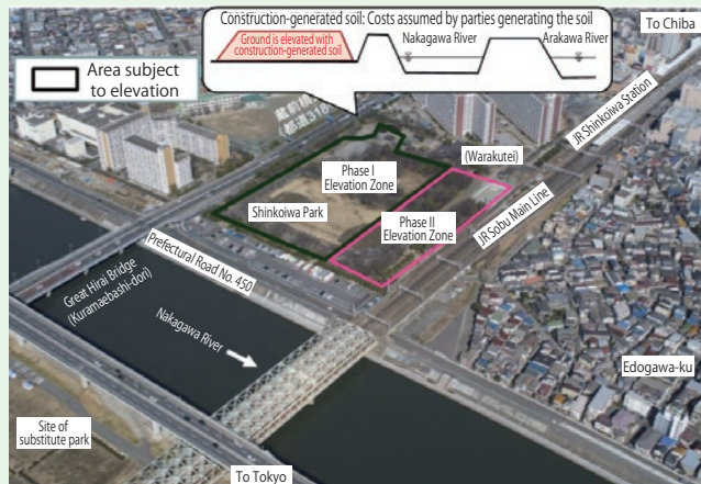
Photo 2: Shinkoiwa Park in Katsushika-ku is elevated.
