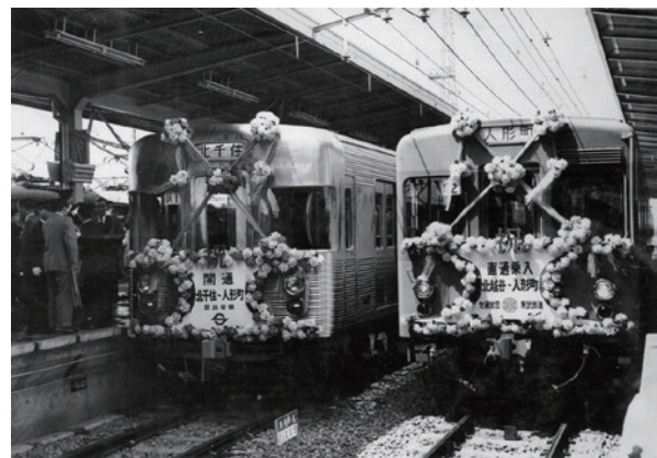
Figure 1-2-29 Opening of Hibiya Line
