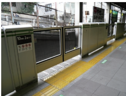
Figure II-7-4-4 Platform door
