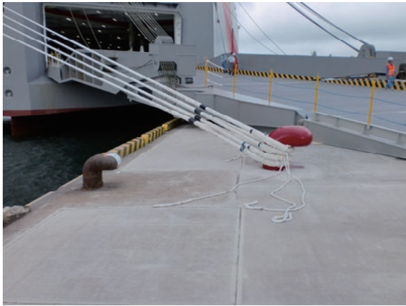
Improved mooring post (right) (The left is the existing mooring post)
