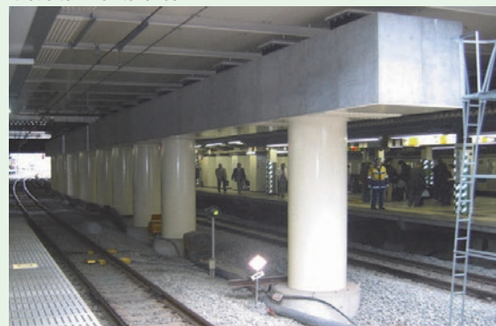
Replaced bridge in 2012
