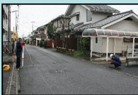
[現況測量の様子]
