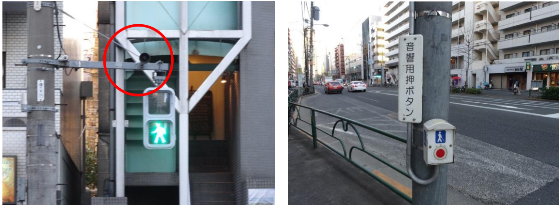
Figure 3.9 Example of Signal for Pedestrians (Left: Speaker, Right: Button for Visually Impaired Persons)
