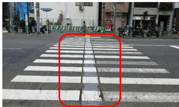
Figure 3.10 Example of Guiding Tactiles on Crossing
