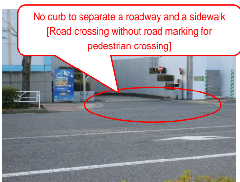
Figure 3.5 Example of Road Crossing without Road Marking for Pedestrian Crossing
