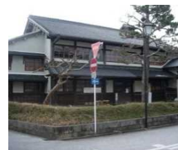
After repairs (current state)
