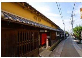
Traditional townhouse transformed into a restaurant
