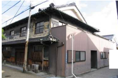
【Restoration/repair of a traditional building】
