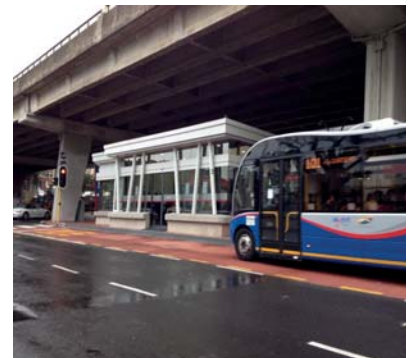
MYCITI BUS AND FEEDER STATION, GARDENS
