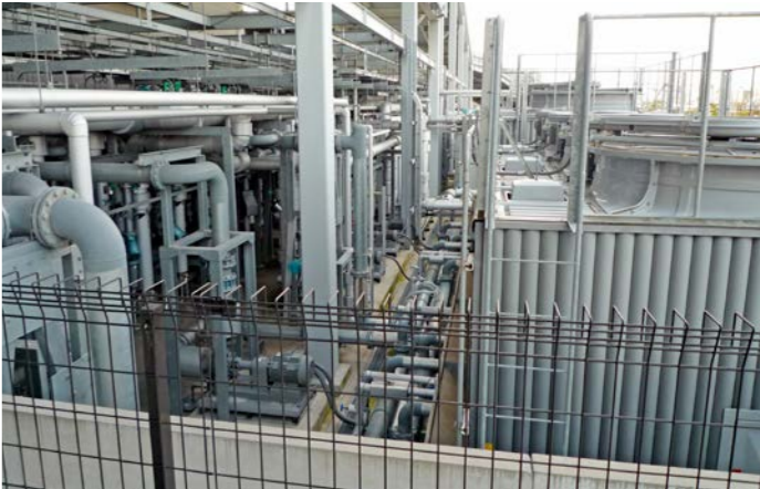
System harvests heat from reclaimed wastewater
