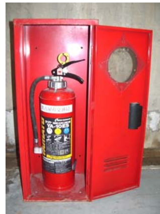
Photo 29.28 Example of fire extinguisher installed independently in a machine room
