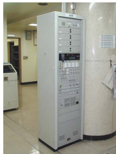
Photo 29.12 Example of public address system
