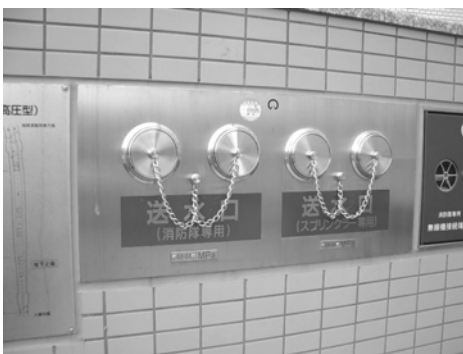
Photo 29.35 Example of water inlet provided by doorway
