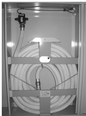
Photo 29.30 Example of easy-to-operate No. 1 hydrant
