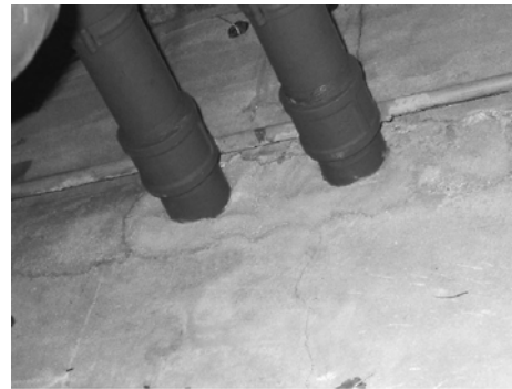
Photo 29.6 Example of treatment of block penetration area
