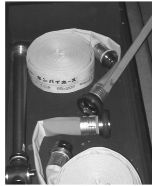
Photo 29.38 Example of water delivery equipment stored in storage box
