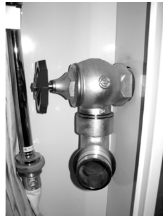
Photo 29.34 Example of water outlet installed in hydrant box
