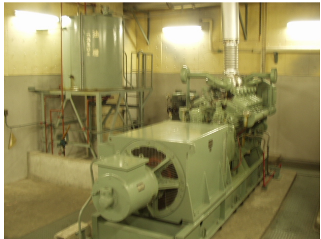
Photo 29.17 Installation example of diesel generator
