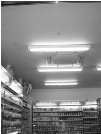
Photo 29.33 Example of sprinkler installed at convenience station store
