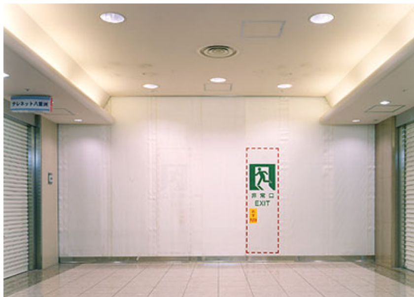
Photo 29.23 Installation example of fire-proof screen
