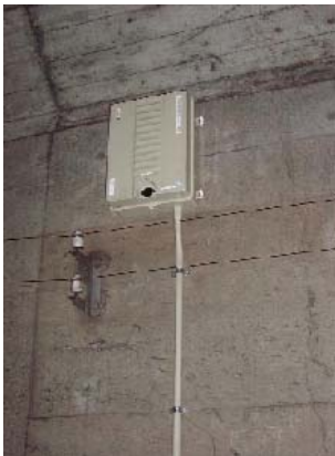
Photo 29.20 Example of PHS Antenna
