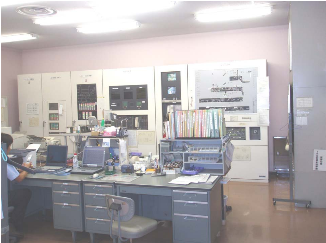
Photo 29.10 Example of using station office as disaster prevention control center
