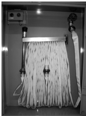
Photo 29.29 Example of No. 1 hydrant
