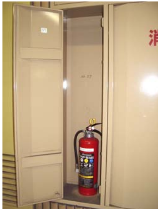
Photo 29.27 Example of fire extinguisher installed side by side with Indoor fire hydrants box
