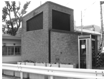
Photo 29.39 Example of water outlet of Internal piping for distributing water for fire fighting between stations on ventilation tower between stations
