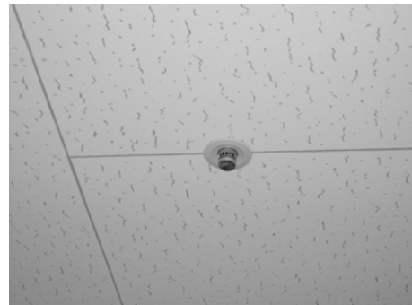
Photo 29.32 Example of sprinkler head
