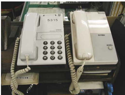
Photo 29.11 Railway telephone (left) Dispatcher telephone (right)
