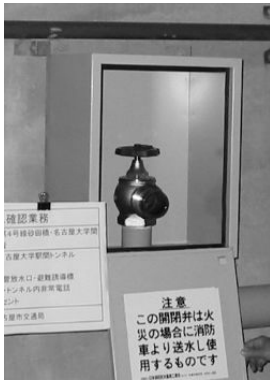
Photo 29.37 Example of water outlets between stations
