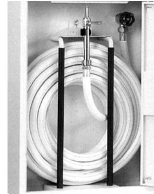
Photo 29.31 Example of No. 2 hydrant
