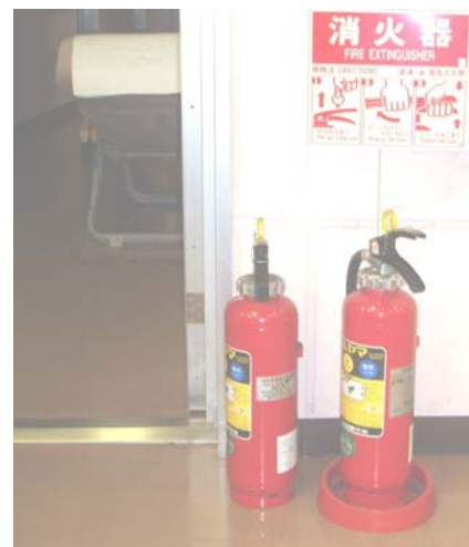
Photo 29.15 Example of fire extinguisher
