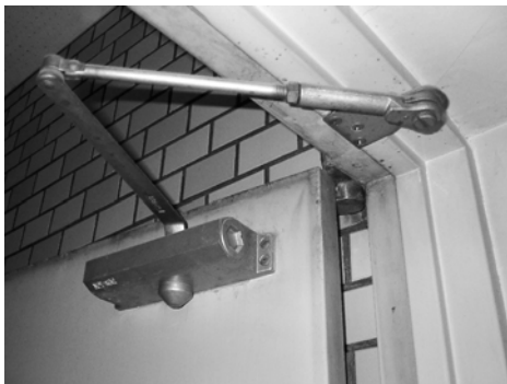
Photo 29.5 Example of automatic closing appliance (door closer)
