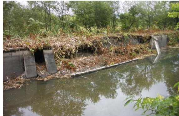
Collapse of the wall at "Hokkai canal"
