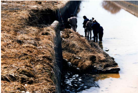
Collapse of the wall at "Hokkai canal"
