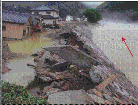
Damage from typhoon No.9 in the Sayo River in 2009
