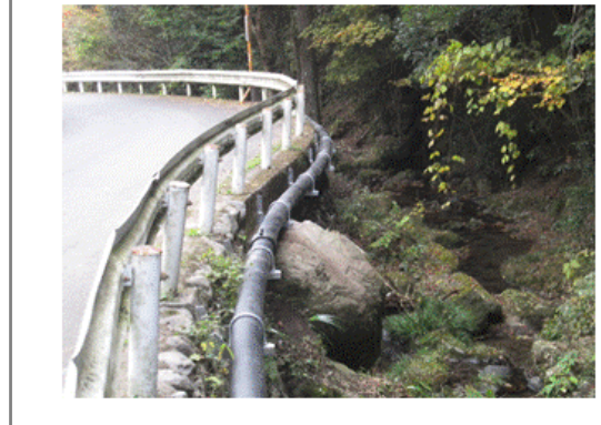
Example case of social experiment (Quick piping (open piping): Hinohara Village in Tokyo)
