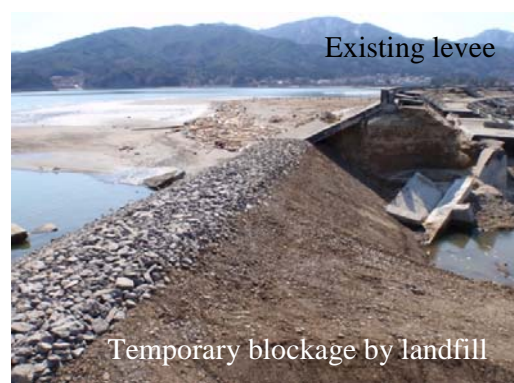
Temporarily reconstructed (Apr. 5)
