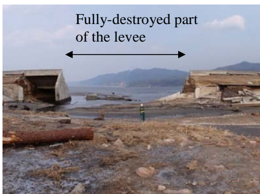
Immediately after the earthquake (Mar. 18)
