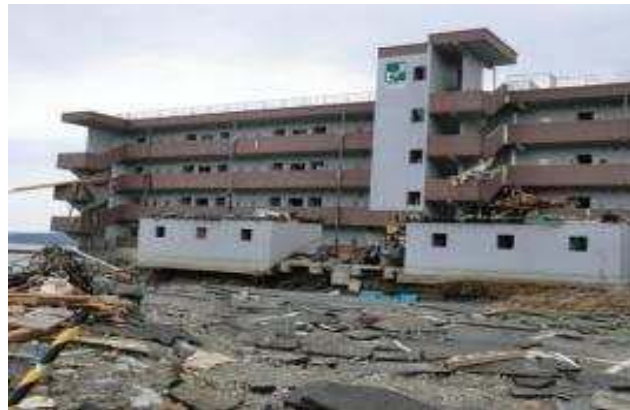
Tsunami Evacuation Building in Sanriku Town, Miyagi
