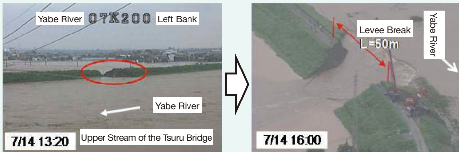
Levee Break Condition of the Yabe River of the Yabe River System
