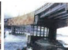
1991 (26 years): Two new columns erected to provide a load-bearing capacity
