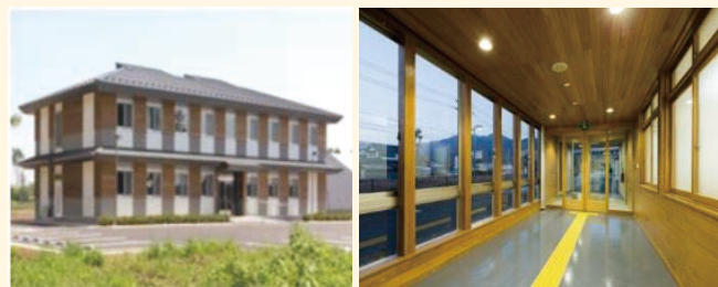
Graphic II-8-1-5 Examples of the use of wood in government buildings
