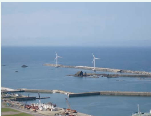
Offshore wind power at Hokkaido Setana Port (Two 600kW turbines)
