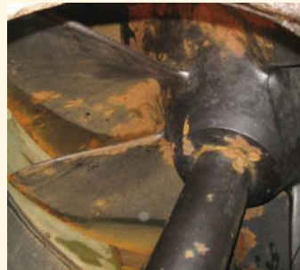
Pump facility impeller
