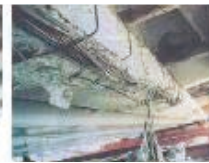
1991 (26 years): Ruptures in the main girder PC steel stock
