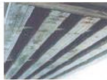
1980 (15 years since construction): Cracks and rust fluid on the bottom face of the main girder
