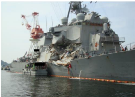
Outside damage ①
