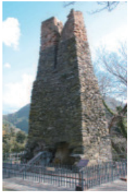
Hagi reverberatory furnace
