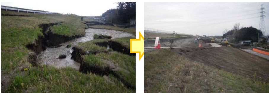
Emergently recovering the most important dike to protect the Capital Area
