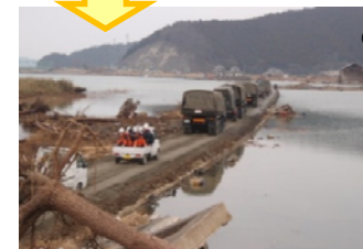
Completed on 14 March
