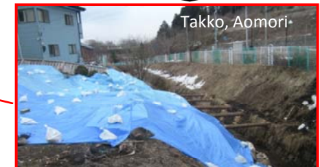
Takko, Aomori Emergency measures have been taken based on the inspection results.
