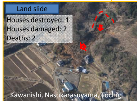
Land slide Houses destroyed: 1 Houses damaged: 2 Deaths: 2 Kawanishi, Nasukarasuyama, Tochigi
