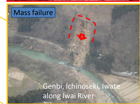
Mass failure Genbi, Ichinoseki, Iwate along Iwai River
