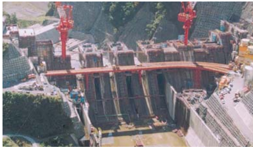
flood control (Dam)
