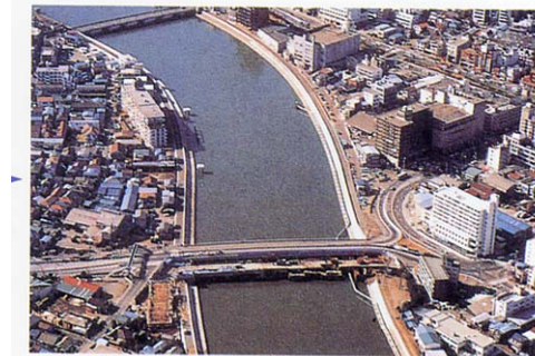
River improvement of Tsurumi river
