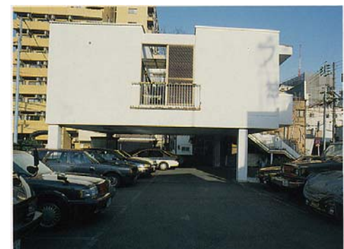
Adopting pilots to prevent damage to buildings during a flood
