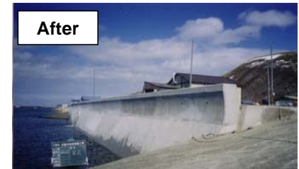
Rehabilitation of aging revetment by setting up anterior wall
