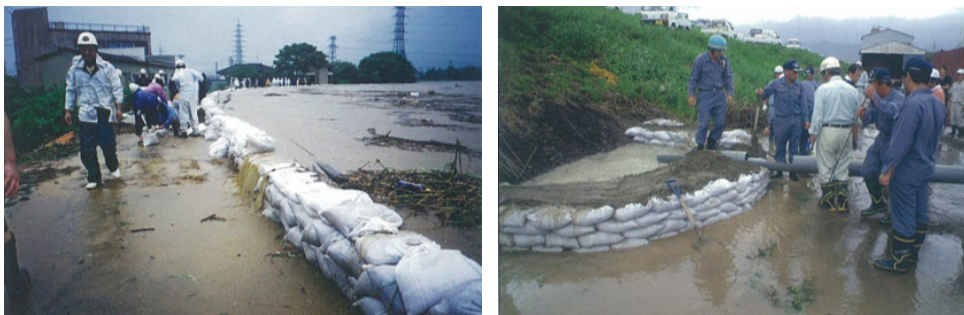
Figure3-13 Flood protection works by flood fighting teams
