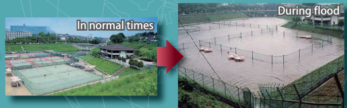
Stormwater storage facilities that are used as tennis courts in normal times (Tsurumi River Basin, Japan)
