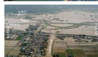
Inundation of National Highway R34 in July 1990 Levees and high-standard roads are free from inundation
