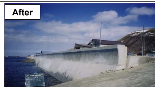
Rehabilitation work by widening of the protection
