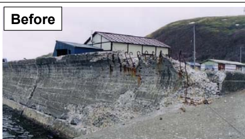
Deteriorated concrete of aging shore protection work
