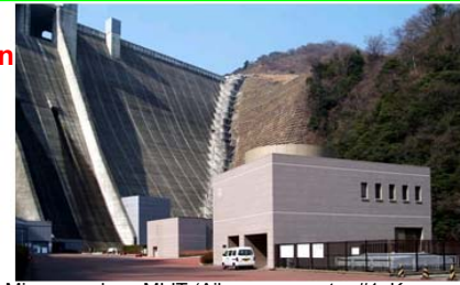
Miyagase dam, MLIT (Aikawa generator #1, Kamagawa)
