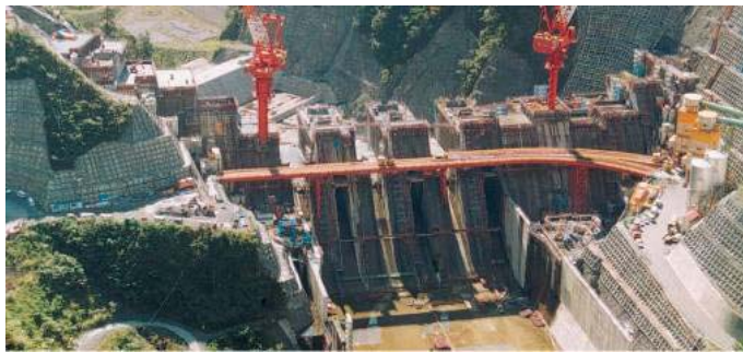
Floodwater regulation structure (Dam)
