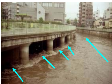
Floodwater regulation structure (Underground regulation pond)
