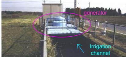
Small-scale generator for agricultural gate operation
