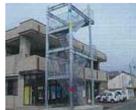
Katahama community disaster prevention center (Sagara, Shizuoka)
