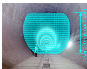
Floodwater regulation structure (Underground regulation pond)
