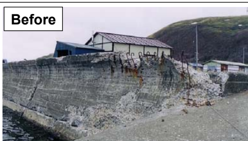
Deteriorated concrete of aging shore protection work
