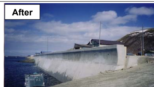
Rehabilitation work by widening of the protection
