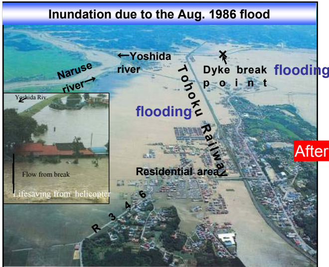
Due to 4 break points, 3,060ha was flooded, 1,510 houses were flooded above the floor level, and some parts of the area stayed under water up to 12 days.
