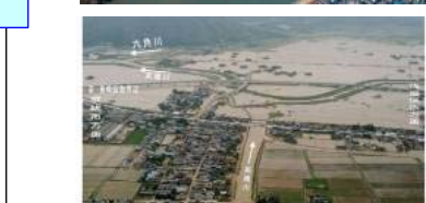
Inundation of National Highway R34 in July 1990 Levees and high-standard roads are free from inundation
