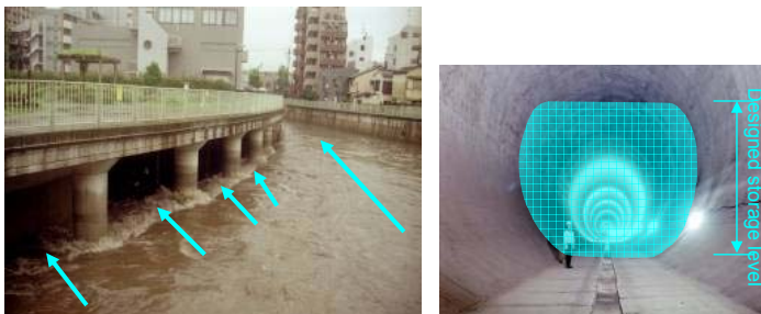
Floodwater regulation structure (Underground regulation pond)
