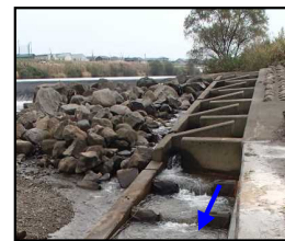
左岸魚道改修前 (H26)
