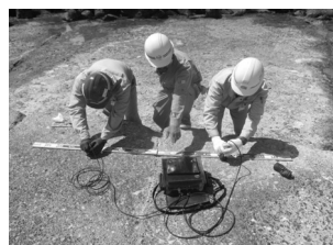
護岸の点検・補修
