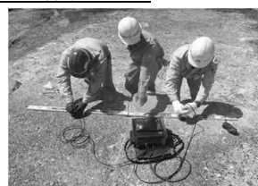
護岸の点検・補修
