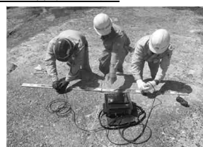
護岸の点検・補修
