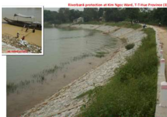
Thirdly, monitor and maintain the river and the structure.
