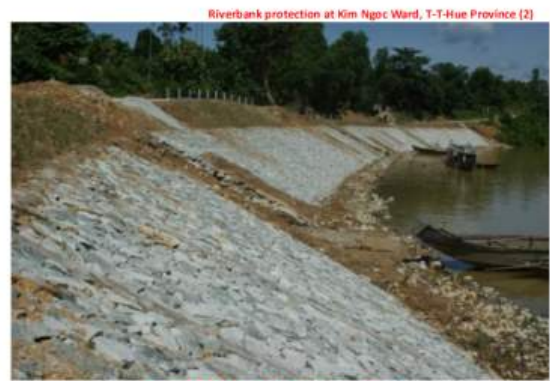
Secondly, build the protection.
