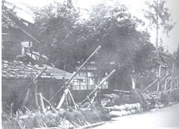
Kawakura skeleton works placed in front of the village for protection from the flood of 1942
