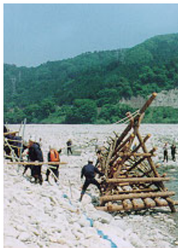
Skeletons assembled during a recent flood-fighting drill
