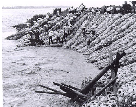
Flood fighting during the flood of 1959 (skeletons and bamboo gabions)
