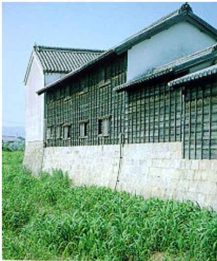
The surrounding wall, made of locally "blue stone," looks like a castle wall.
