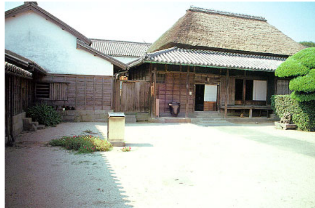
The main building viewed from inside the premises.
