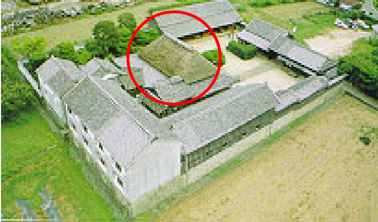
An overview of mizuya surrounded with a wall. The main building shown in the center of the photograph has a thatched roof, which is designed to float on water in the event of an extreme flood.
