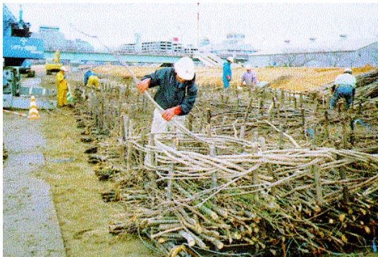
Weaving a fascine mattress
