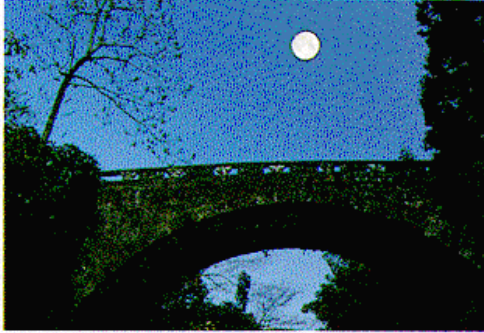
1) 48 Nagayama Bridge (Kikuchi City): prefecture-designated important cultural property; the original bridge built in 1824, the new bridge built in 1878; mason for the original bridge: Kosaka Kangoro, mason for the new bridge: Hashimoto Kangoro; length: 61.00 m, width: 4.50 m, height: 16.00 m, span length: 20.60 m, rise: 7.90 m
