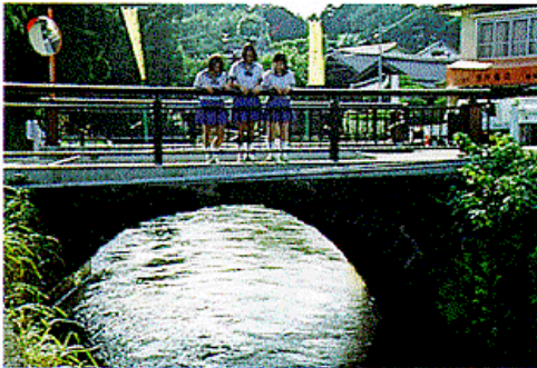
3) 67 Jizo Bridge (Otsu City): town-designated cultural property; completed in ca. 1814; mason: Kantaro (probably); length: 7.50 m, width 4.35 m, height: 3.65 m, span length: 6.00 m, rise: 3.00 m
