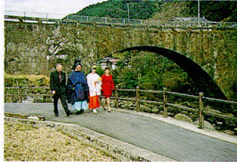
2) 53 Tatekado Bridge (Kikuchi City): prefecture-designated important cultural property; completed in 1860; mason: Uichi; length: 75.00 m, width: 3.60 m, height: 11.40 m, span length: 21.70 m, rise 8.60 m
