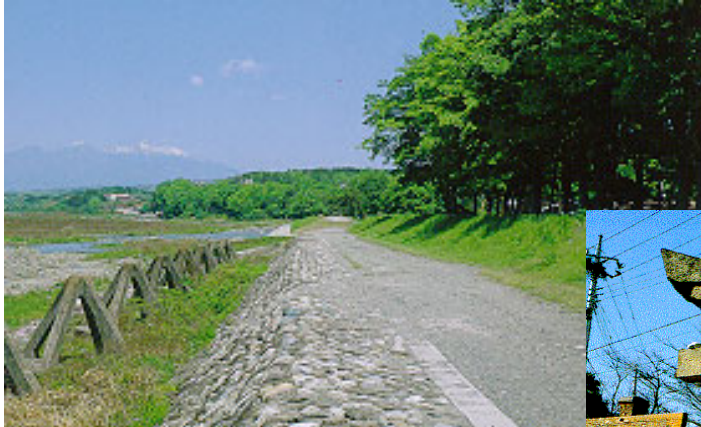
Present Shingen Levee (continuous levee)
