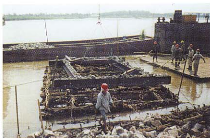
Placing the H-shaped steel frame weight to submerge the groin Soda-mattress
