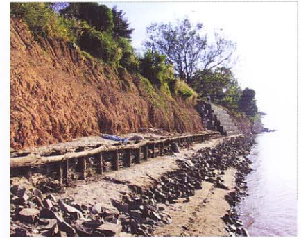
Eleven months after the pilot construction (February 2002)
