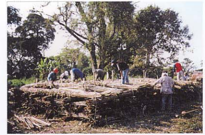
Linking upper and lower lattices
