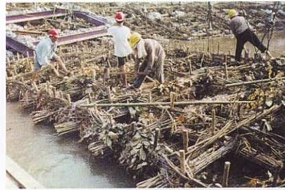
Final-driving of short piles immediately before the installation of Soda-mattress
