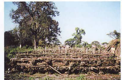
Assembled Soda-mattress units
