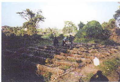
Framing lower lattice with bundled fascines
