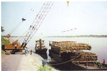
Loading Soda-mattress onto the material barge
