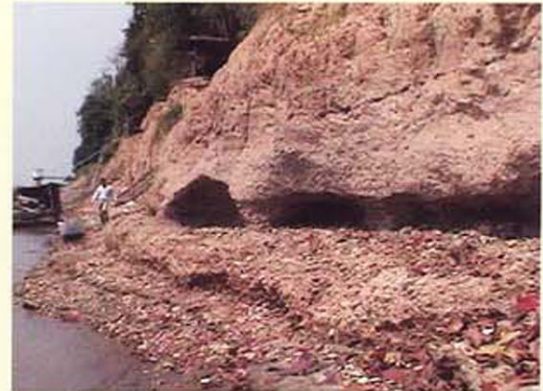
Notches formed around the foot of the riverbank at the pilot project site (March 2000)
