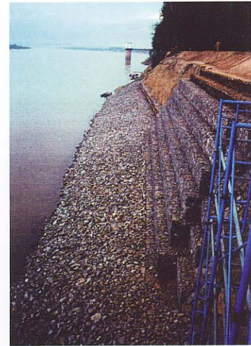
Immediately after the pilot construction (March 2001)
