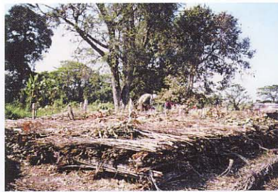
Spreading 3 layers of loose fascine
