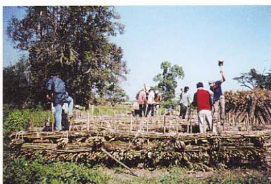
Half-driving of short piles
