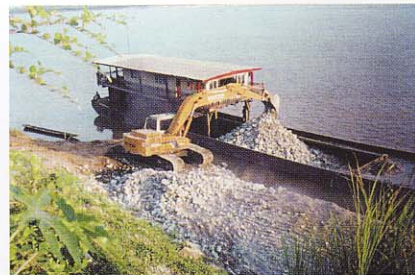
Loading riprap onto the material barge with a backhoe
