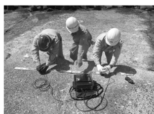
護岸の点検・補修
