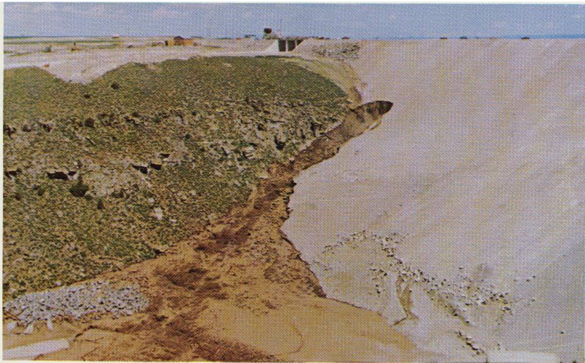
Fig. 2-10. Dozers lost in hole. About 11:20 a.m. June 5, 1976.
