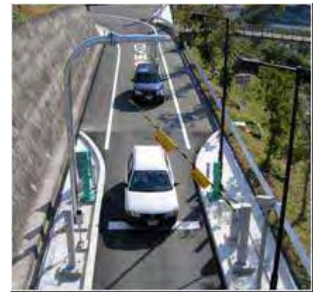
Fig. Smart interchange at Yoshinokawa Service Area
