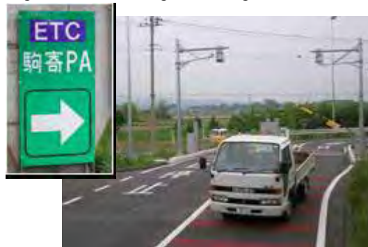
Fig. Smart interchange at Komazaki Parking Area
