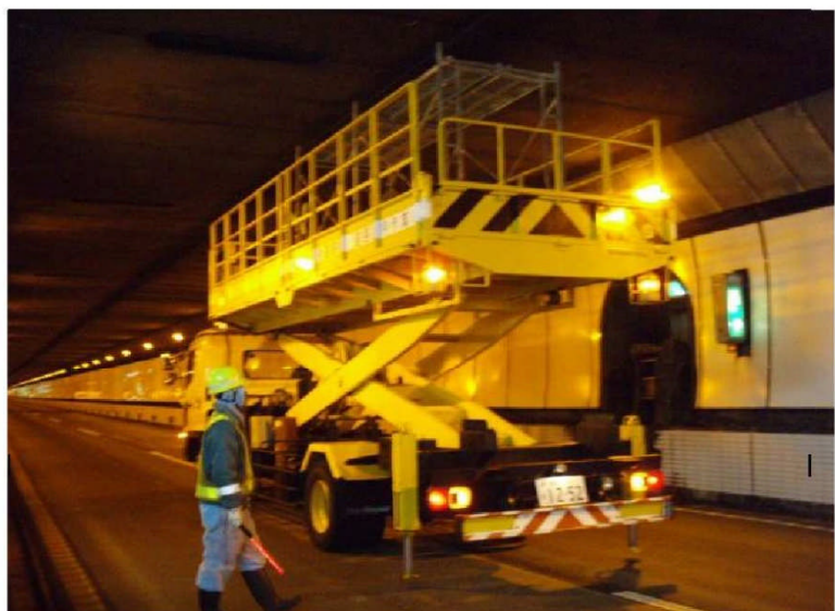
③ 点検天井板直下リフト車配置
